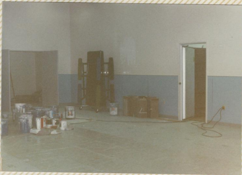
Still working on the new cafeteria.
