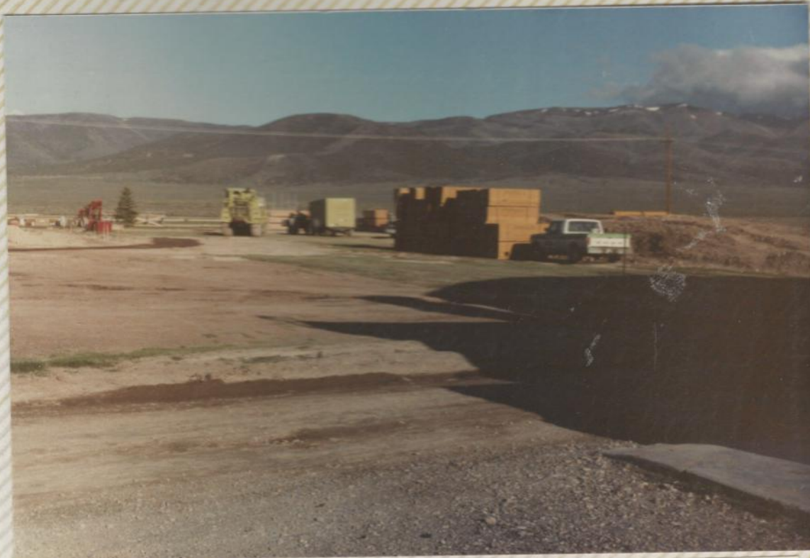
Neddo Construction (green) looking east toward "R"
