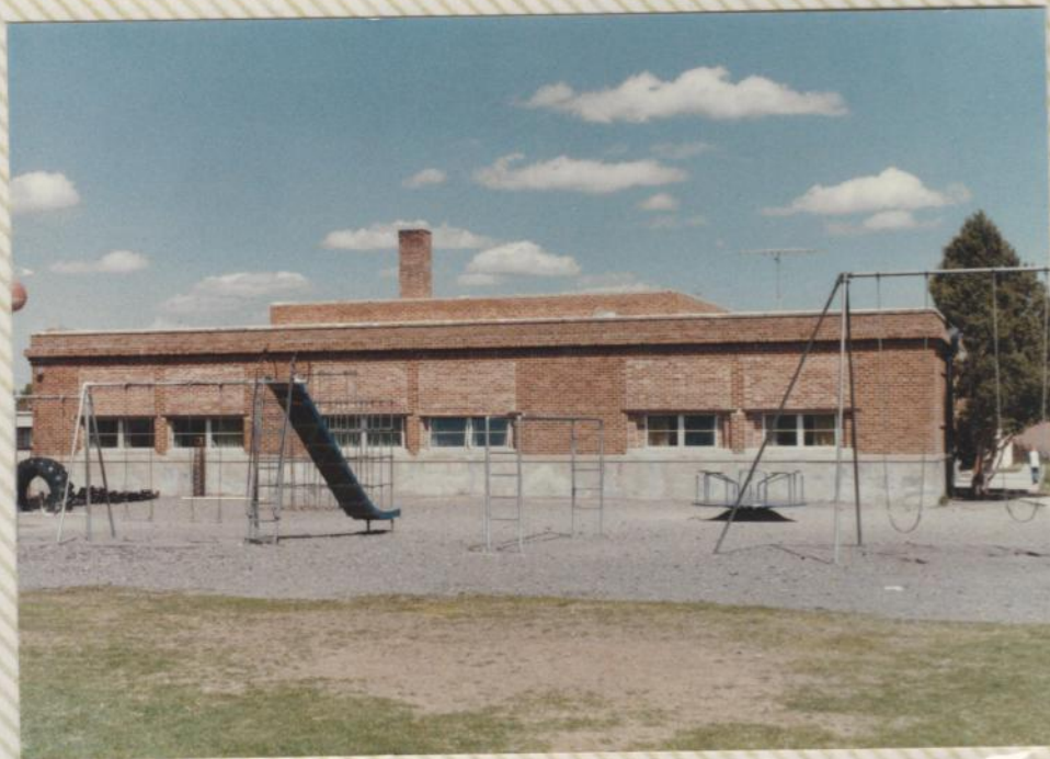
MALTA ELEMENTARY --MAY 1989 (South-east side)
