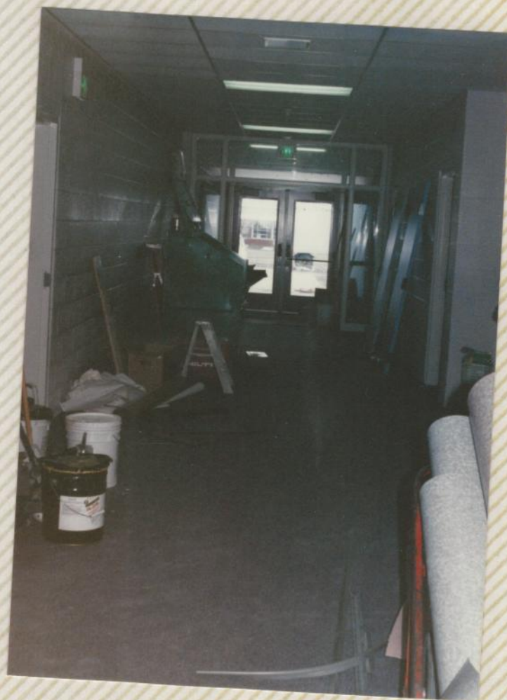
Hall in front of locker rooms-still a ways to go.
