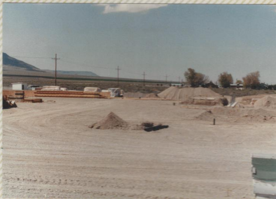
NEW SCHOOL SITE--MAY 1989 (looking north)
