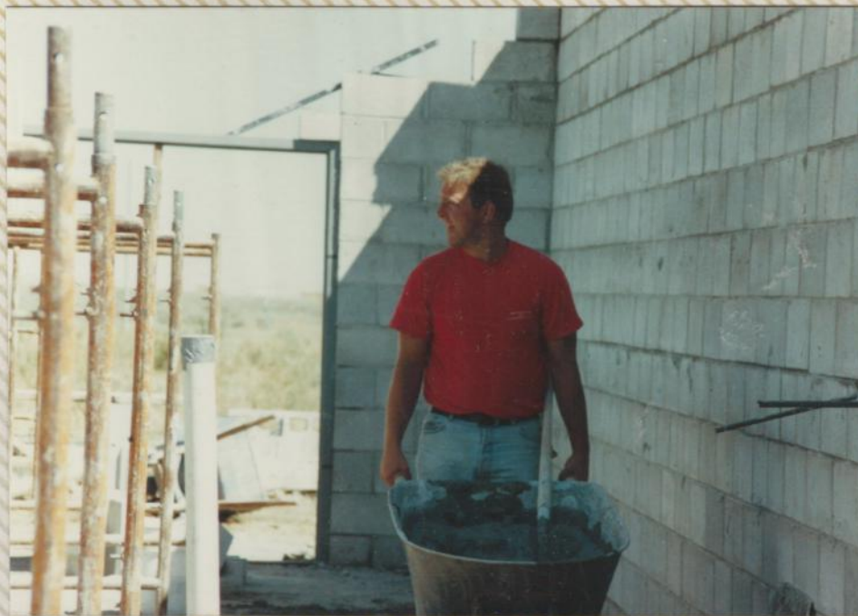
Richins "Pumping Cement"
